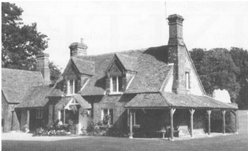
The Castle Cottage belongs to the Duchy of Cornwall.
