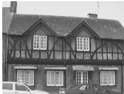
An example of a building within the conservation area with plastic windows.
