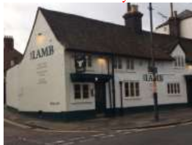
The Lamb, 277 High Street Refurbishment & works to rear yard etc
