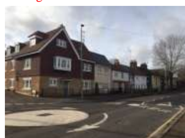
Corn Mill Ct, 9-13 High St & Swing Gate La Demolition etc for 11 new dwellings# through conversion and new build
