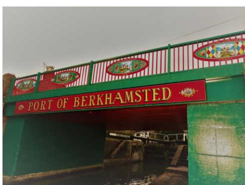
Ravens Lane bridge
