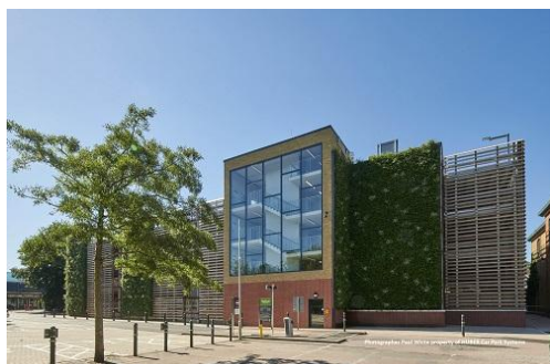
Multi-storey car park
