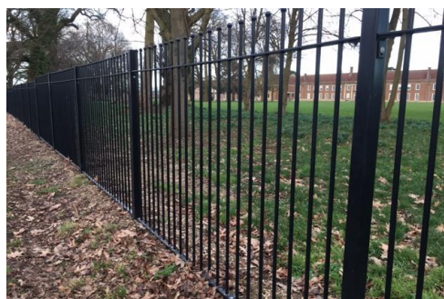
Railings at the front of Ashlyns School
